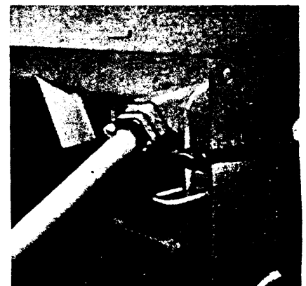
6. Lengthen brace and install bolts. Tighten bolts to 280 \pm 20 lb. ft. ( 38,75 \pm 2,75 mkg). Lubricate ball and socket.
