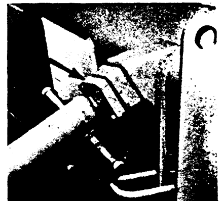
3. Lengthen brace. Install and tighten bolts evenly.
